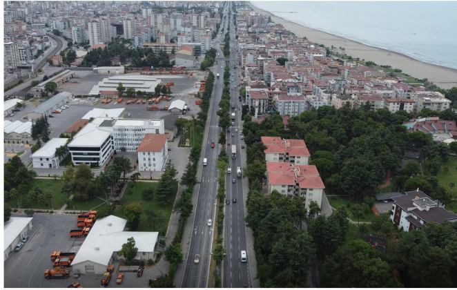
Fig. 2. Drone image of the area containing the intersections.
